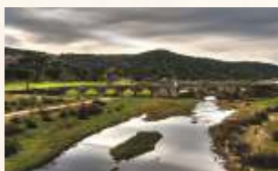
Bridge over the Almonte river
