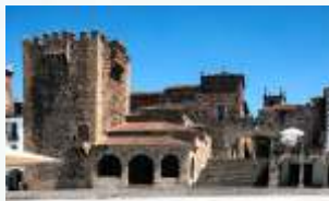
Torre de Bujaco (praça Mayor)
